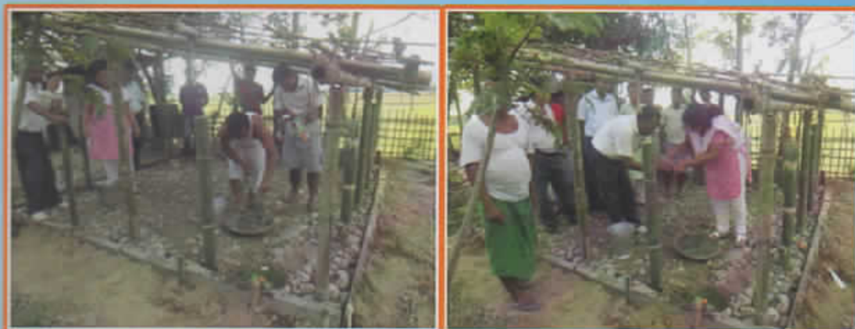
Starting of construction works of pigsty at Solokhoni village
